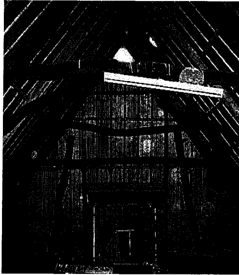
Some of the 160-plus-year-old beams and rafters, which appear to have been nothing more than roughly hewn large tree branches, have survived to this day.
